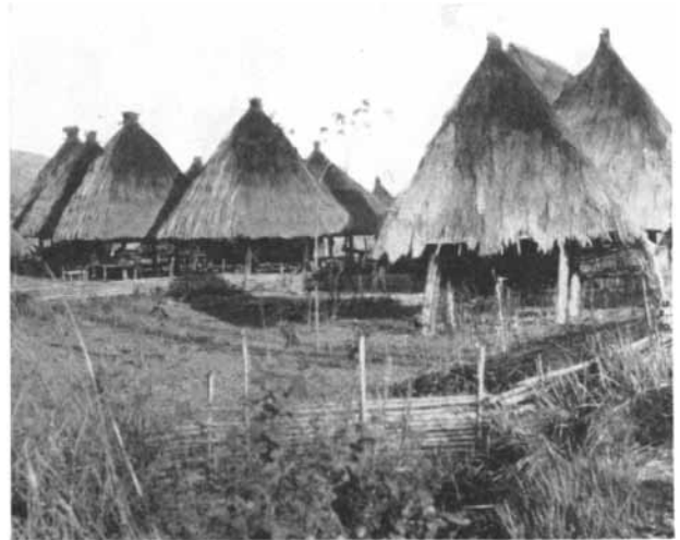
SOUTH SEA VILLAGE on Alor Island near Borneo shows light parasol construction so admirable for regions of heavy rainfall.
