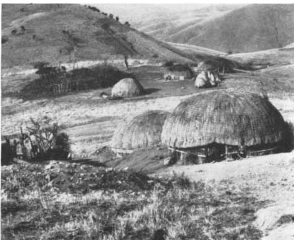
ZULU KRAAL in Union of South Africa answers climate problem with thatched huts built on woven framework of light branches.
